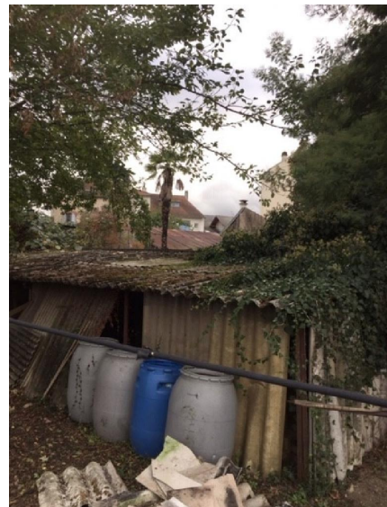
COUVERTURE PLAQUE FIBRE CIMENT
