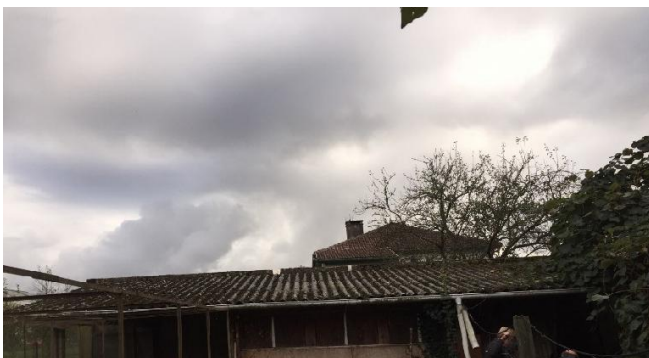
COUVERTURE PLAQUE FIBRE CIMENT
