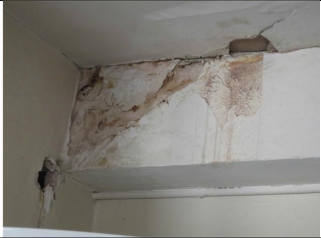
A photograph showing significant water damage on a white ceiling. The damage is characterized by large, irregular brown stains and areas where the ceiling material has been removed or is peeling away, revealing a darker substrate. The damage is concentrated in the upper part of the frame, near the corner of the room. |       |
