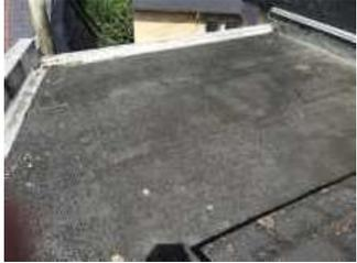
A photograph showing a flat roof surface covered in dark, textured bituminous material. A concrete curb is visible on the left side. |
